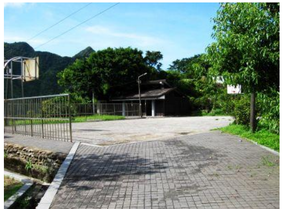
Area of the old unused basketball court at the back of the park before the construction of Phase II
